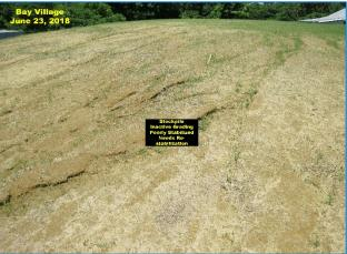
Grass is present in both photos above but is far below the 95% groundcover required by Standard & Specification B-4. And while straw mulch is commonly seen on most construction sites, the protective layer tends to be far below the *complete blanketing* needed to obscure underlying soil from view as required by Standard & Specification B-4-3. Failure to meet both standards results in the erosion seen in the photo to the right and unnecessary pollution of nearby waters.
