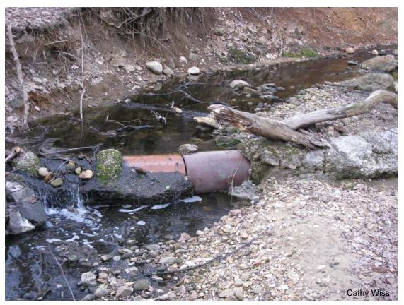
(An eroded and cracked sewer pipe that has been repaired more than once)
